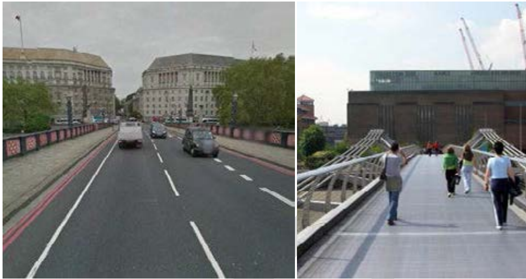
Figure 22 – Lambeth Bridge and pedestrian bridge (Millennium)
